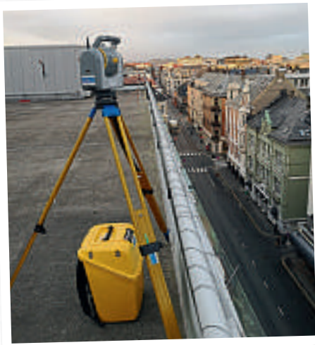
The SX10 scans all of the roof's features including picnic tables and benches, utilities, air vents and fencing along the external edges. © Geomatikk Survey
